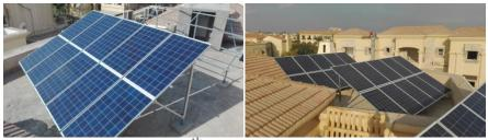
4. Gardenia Project, 6<sup>th</sup> October, Egypt On Grid System On Grid (Fronius) 12.5 KW Components: PV Solar Modules: Jurawatt Poly 250 WP On Grid Inverter: Fronius Symo 12.5 KWP
