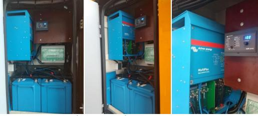
MCV Bus Project (Automotive) Salhya, Egypt Bus Backup System Off Grid (Victron) 5 KW Components: Off Grid Inverters: Victron Multiplus 5 KWP Batteries: Victron Lithium 200 Ah x 2
