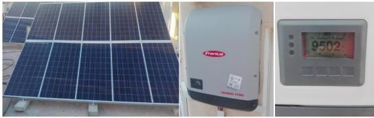
5. Villa 15 Marina 23 Project, North Coast, Egypt On Grid System On Grid (Fronius) 12.5 KW Components: PV Solar Modules: Jurawatt Poly 250 WP On Grid Inverter: Fronius Symo 12.5 KWP
